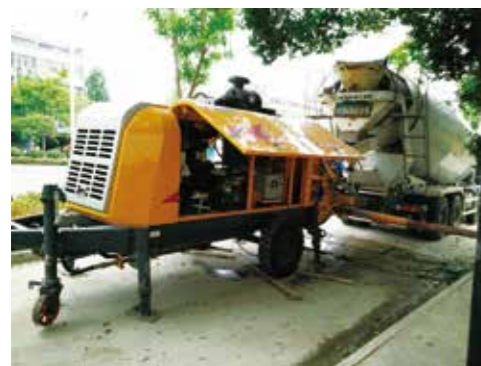
HBT6013V 江苏徐州 HBT6013V trailer-mounted concrete pump in Xuzhou, Jiangsu
